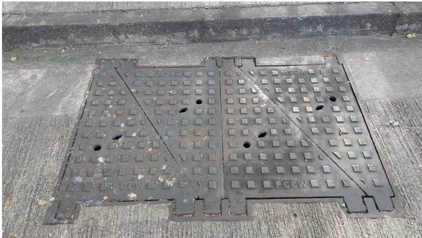
Photo No. 9e - (Carriageway Joint Box – Cast Iron Type) No. of Cover: 4
