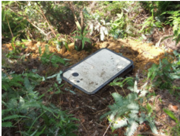
Photo No. 11a - (Joint Box – Plastic Type) No. of Cover:1
