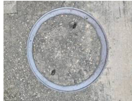
Photo No. 8c - (Carriageway Manhole – Concrete/Cast Iron Type) No. of Cover: 1
