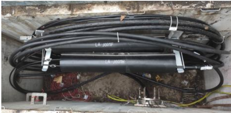
Photo No. 5a - (Cables) Inside Jointing Chamber
