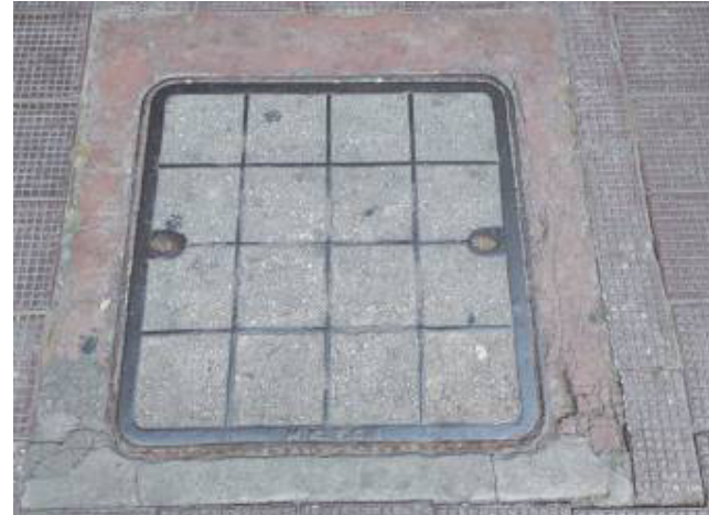
Photo No. 8a - (Footway Manhole – Concrete/Cast Iron Type) No. of Cover: 1
