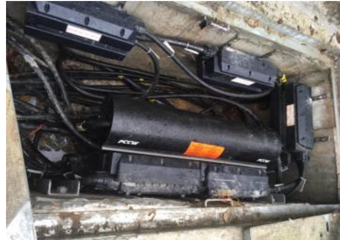
Photo No. 6b - (Cable Joint) Inside Jointing Chamber
