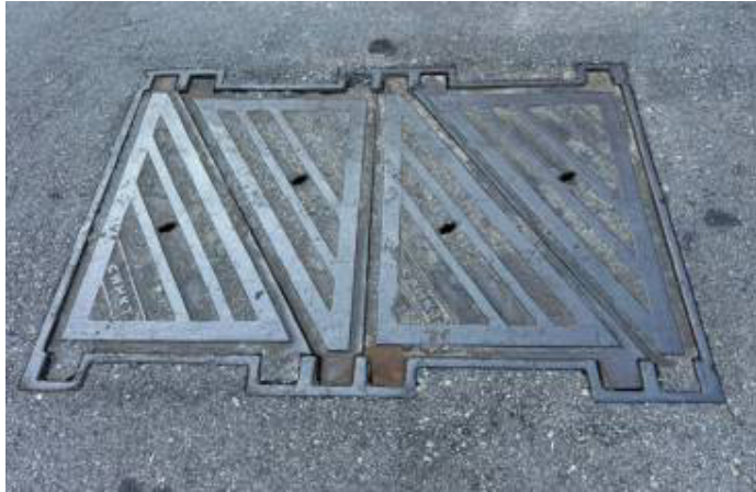
Photo No. 9c - (Carriageway Joint Box – Cast Iron Type) No. of Cover: from 4
