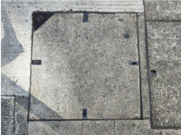
Photo No. 7e - (Footway Manhole – Concrete Type) No. of Cover: 1
