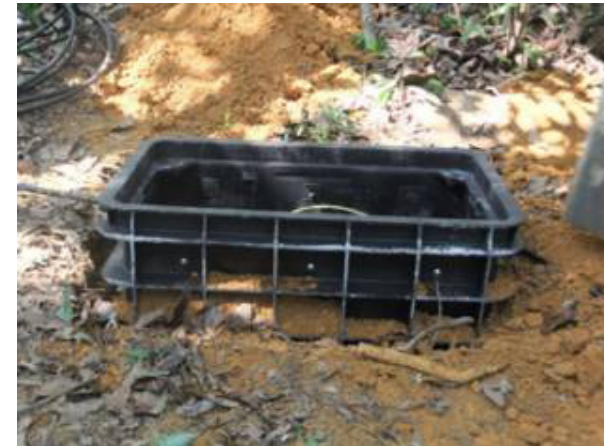
Photo No. 11b - (Joint Box – Plastic Type) No. of Cover:1
