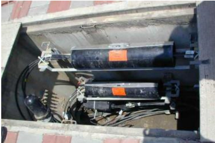
Photo No. 6a - (Cable Joint) Inside Jointing Chamber
