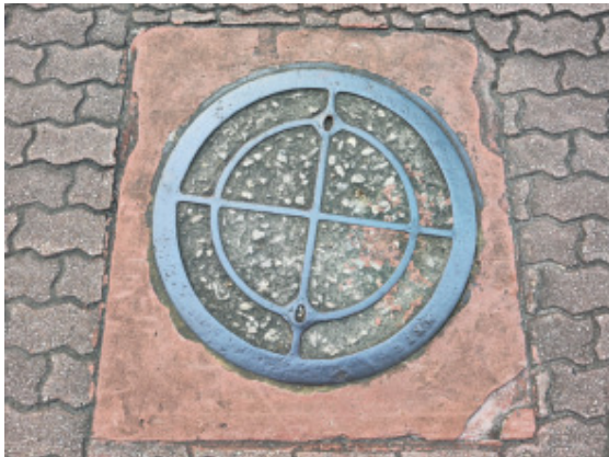
Photo No. 8b - (Carriageway Manhole – Concrete/Cast Iron Type) No. of Cover: 1
