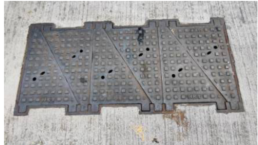
Photo No. 9f - (Carriageway Joint Box – Cast Iron Type) No. of Cover: 6
