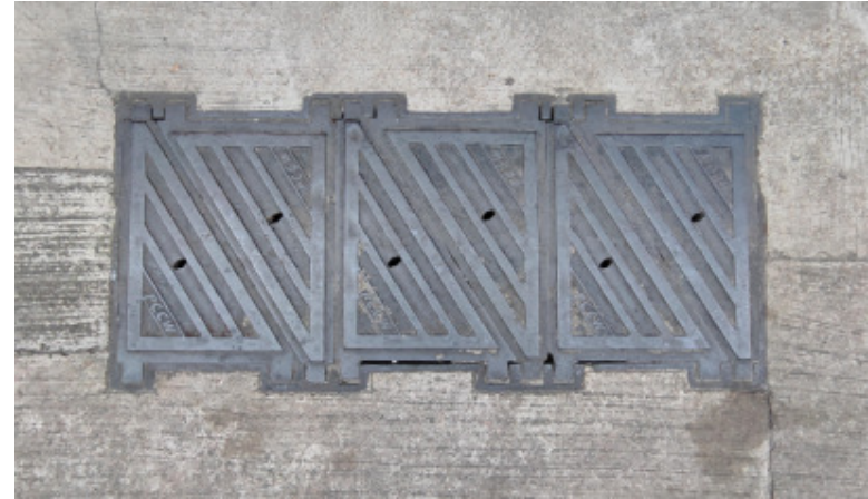
Photo No. 9d - (Carriageway Joint Box – Cast Iron Type) No. of Cover: 6
