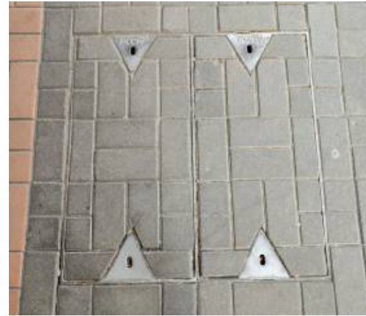
Photo No. 10f - (Footway Manhole – Recessed Type) No. of Cover:2
